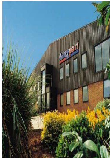
Glazpart's state of the art factory and warehouse facility in Banbury, Oxfordshire.
